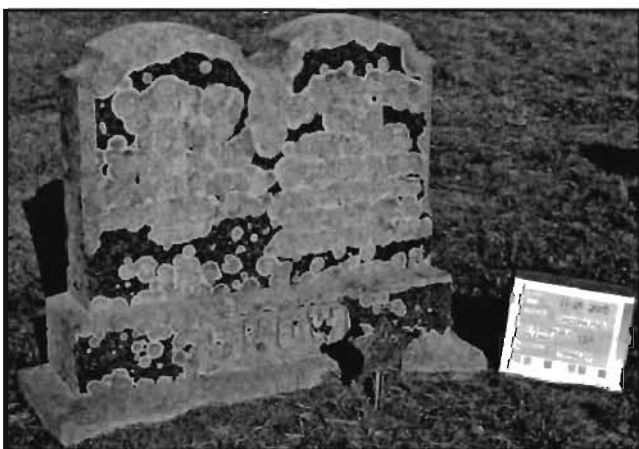
Granite die on base showing severe growth of crustose lichens over both unpolished and polished surfaces.
