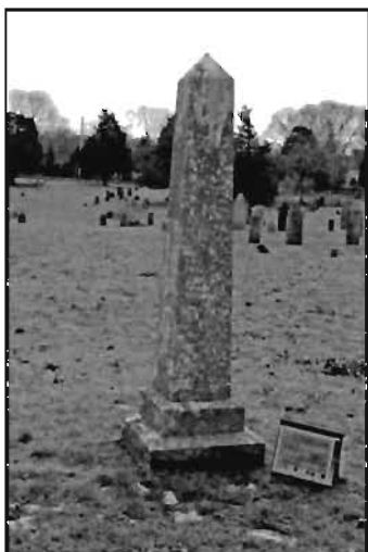
Marble obelisk showing moderately severe growth of crustose lichens.
