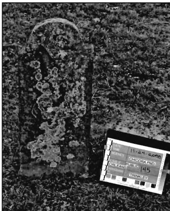
Sandstone headstone showing both crustose and foliose lichen. Although much of the face has spalled off, the small amount left is unreadable because of the lichen deposits.
