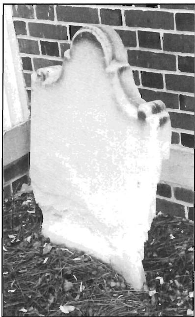
Severe efflorescence with stone loss.
