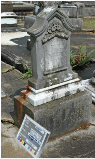
Before Treatment— note the corrosion staining on the left side.
