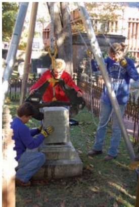
Although an aluminum tripod such as this can make moving heavy monuments easier, it also requires additional safety practices.
