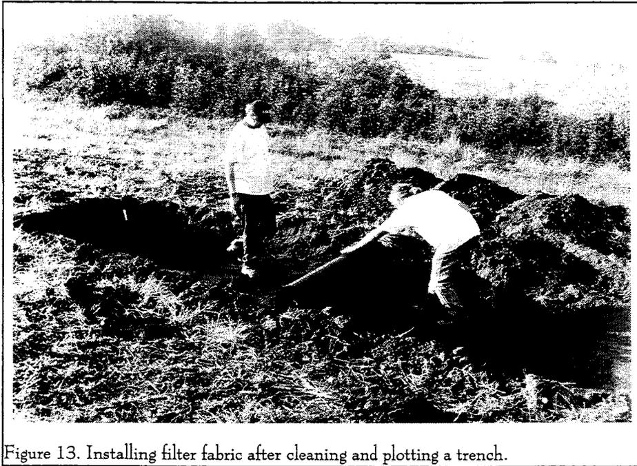
Figure 13. Installing filter fabric after cleaning and plotting a trench.
