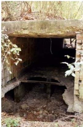
View of drier interior, looking southwest. The flue area is shown under the kiln.
