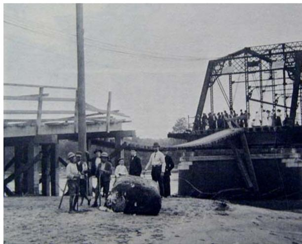
Figure 21. View of the 1891 Thirteenth Street bridge damaged during the 1929 flood (adapted from Rosson 1980:209).
