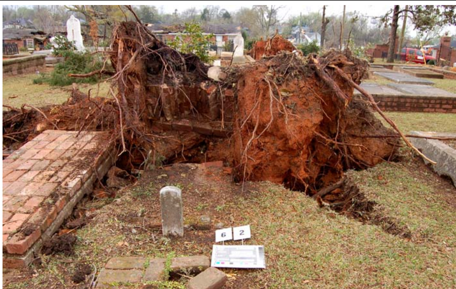
Figure 5. Example of vault damage requiring archaeological investigation. The open vault should also be secured prior to conservation treatment to prevent looting, desecration, or vandalism.
