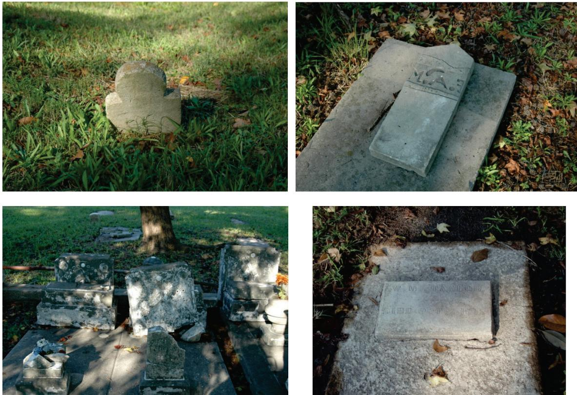
Figure 43. Examples of cast stone (Portland cement) monuments. These examples show a variety of designs, cast inscriptions, inclusions, and use of whitewash.
