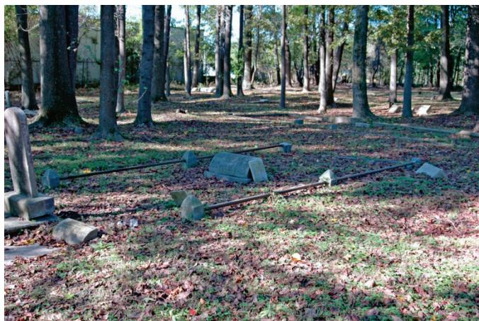
Figure 44. Examples of ironwork in the cemetery complex. Upper photo shows a remnant portion of a “hairpin” section. Middle photo shows a remnant corner post. Lower photo shows a gas pipe fence set in low concrete posts.
