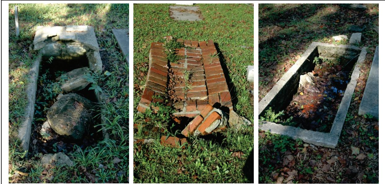
Figure 42. Examples of damaged (or lost) vault tops that should be replaced with new cast concrete slabs.
