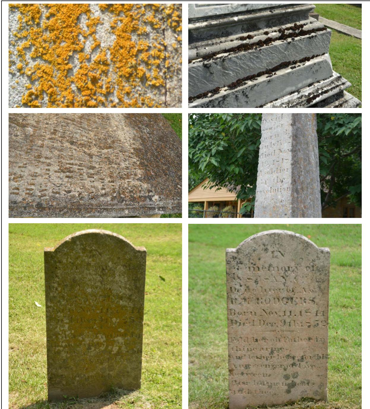
Figure 76. Cleaning issues in the cemeteries. Upper left shows a close-up of lichen on a stone at City Cemetery. Upper right shows a different lichen form at Rest Haven Cemetery. Middle left shows a table tomb harshly cleaned in an effort to read the inscription. Middle right shows an improperly cleaned inscription on an obelisk; the remainder of the monument was left soiled. Bottom shows a stone before and 10 minutes after cleaning with D/2 Biological Solution.
