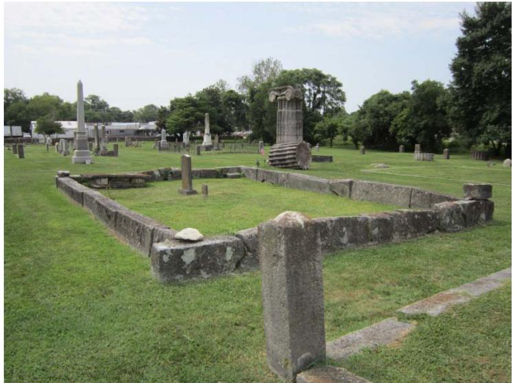
Figure 64. Displaced or damaged curbs and copings. Upper photo shows displaced coping in City Cemetery. Lower photo shows broken and badly displaced wall coping at Rest Haven Cemetery.
