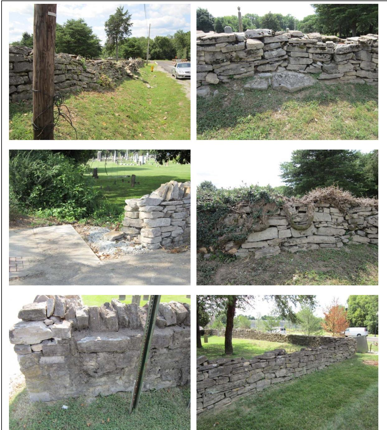
Figure 31. Condition of the stone wall at Rest Haven Cemetery. Upper left shows an overview of damage along the east wall. Upper right shows very poor construction techniques in one area. Middle left shows the terminus of the southern wall without a stroup. Middle right shows vegetation allowed to overtake the wall. Lower left shows the southeast corner with Portland cement repair. Lower right, missing top stones, northeast corner.
