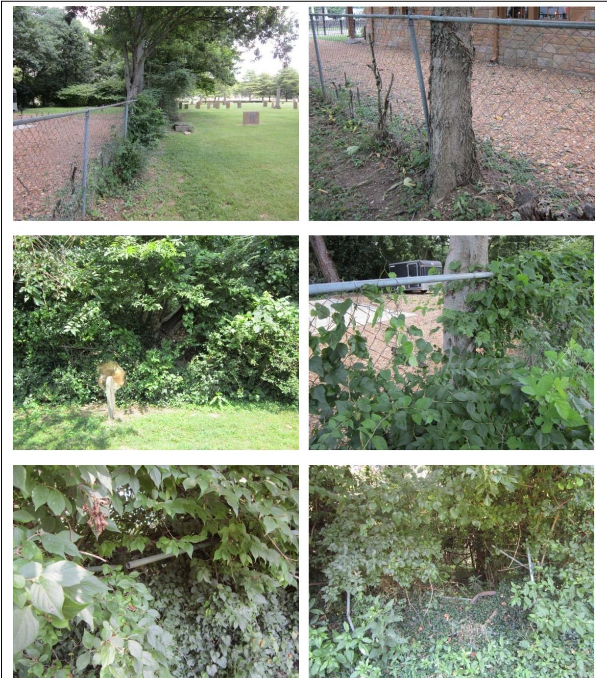
Figure 29. Chain link fence along the north property line. Upper left, vines and other vegetation should be removed from the fence. Limbs from adjoining property should be removed to the property line. Upper right shows a tree grown into the fence. Middle left shows a tree fallen on the fence. Middle right shows a second tree growing into the fence which must also be removed. Lower left shows a damaged and bent top rail. Lower right shows a section of fence that is totally down.
