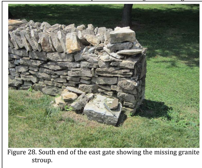
Figure 28. South end of the east gate showing the missing granite stroup.
