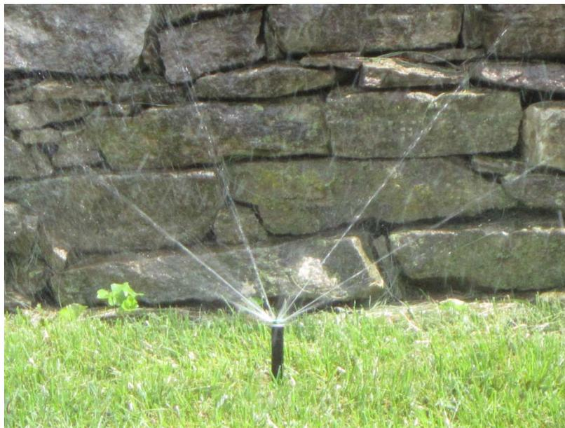
Figure 33. Sprinklers wetting the north cemetery wall should be removed or adjusted to ensure the wall remains dry.
