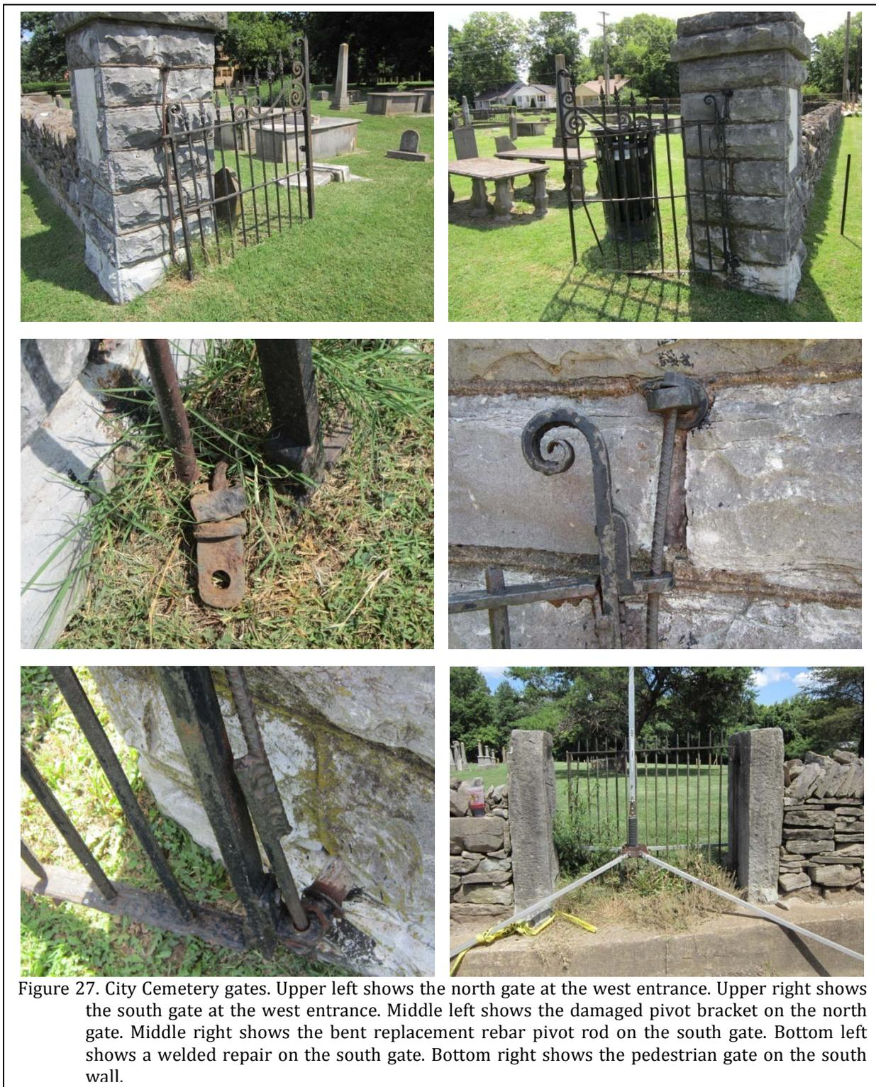
Figure 27. City Cemetery gates. Upper left shows the north gate at the west entrance. Upper right shows the south gate at the west entrance. Middle left shows the damaged pivot bracket on the north gate. Middle right shows the bent replacement rebar pivot rod on the south gate. Bottom left shows a welded repair on the south gate. Bottom right shows the pedestrian gate on the south wall.
