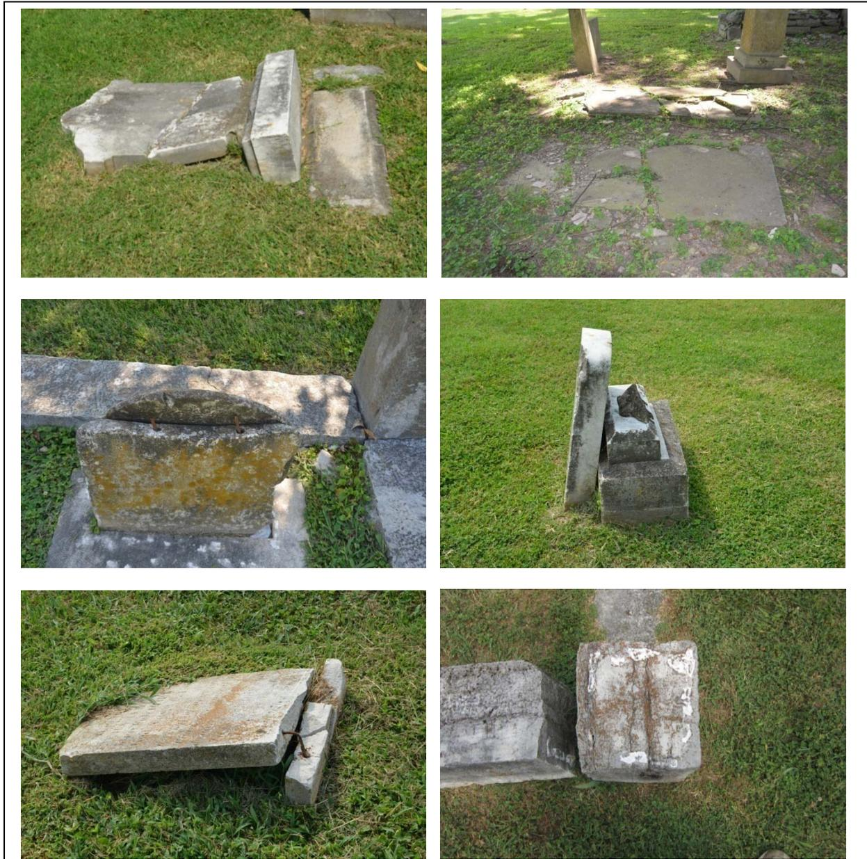
Figure 70. Examples of broken stones. Upper left shows a die on two bases. When the stone fell or was pushed over, the impact of hitting the ground caused the die to break. Upper right shows a badly broken marble ledger. Middle left shows a tab in socket with the die broken and use of ferrous pins in a failed repair. Middle right shows a broken tab in socket. Lower left shows a headstone and use of ferrous pins in a failed repair. Lower right shows a failed simple epoxy repair.
