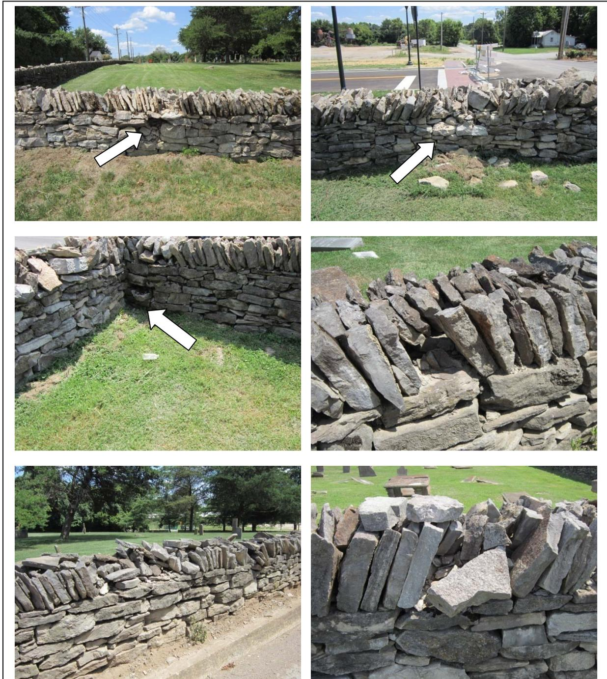
Figure 26. City Cemetery stone wall defects. Upper row shows damage to the eastern wall, exterior (left) and interior (right). Middle left, southeast interior corner showing stone loss. Middle right, south exterior loss of capping stones. Lower left, jumbled and dumped capping stones on the south wall. Lower right, west wall damaged cap.
