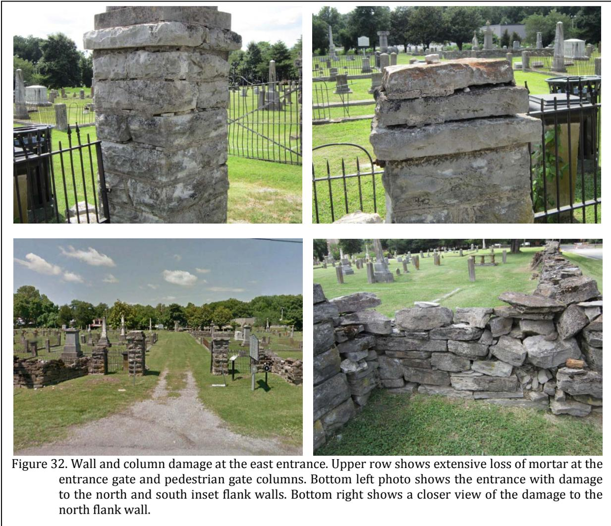
Figure 32. Wall and column damage at the east entrance. Upper row shows extensive loss of mortar at the entrance gate and pedestrian gate columns. Bottom left photo shows the entrance with damage to the north and south inset flank walls. Bottom right shows a closer view of the damage to the north flank wall.
