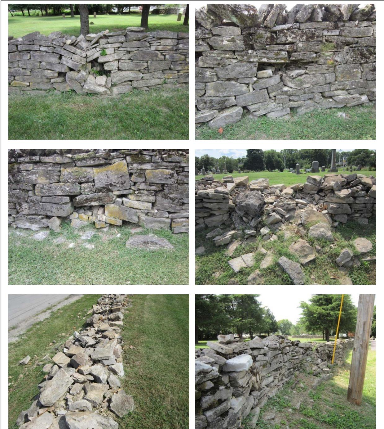
Figure 30. Condition of the stone wall at Rest Haven Cemetery. Upper left shows a slump on the east exterior wall. Upper right shows stone loss and incipient slump on the east wall. Middle left, stone loss with stones partially buried in the soil beyond the wall. Middle right shows more extensive area of wall collapse. Lower left shows total collapse of the wall. Lower right shows bowing of the wall.
