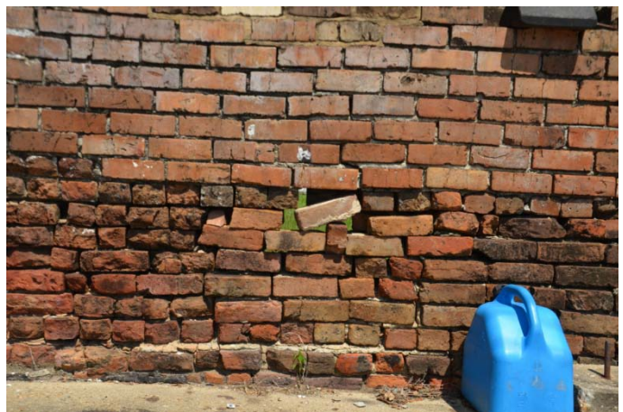
Figure 25. Examples of boundary wall problems. Upper photo shows the exterior of the east wall with multiple repair episodes, none meeting preservation standards. Lower photo shows a portion of the south wall approaching failure.
