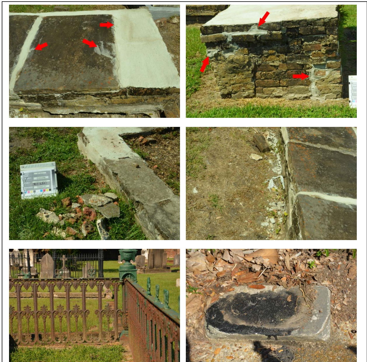
Figure 46. Past repair efforts and work in the Church Street Graveyard. Upper left photo shows mortar smears and a recent shrinkage crack forming (since mortar is not intended to be used as stucco). Upper right photo shows very poor pointing with mortar smeared over the brick, very wide joints, and unfinished joints. Middle left photo shows brick rubble not picked up after repair of corner. Middle right photo shows rubble not collected after repairs. Lower left photo shows one of several fences painted only on the outside. Lower right photo shows where paint was spilled on a footstone with no effort to clean up the spill.
