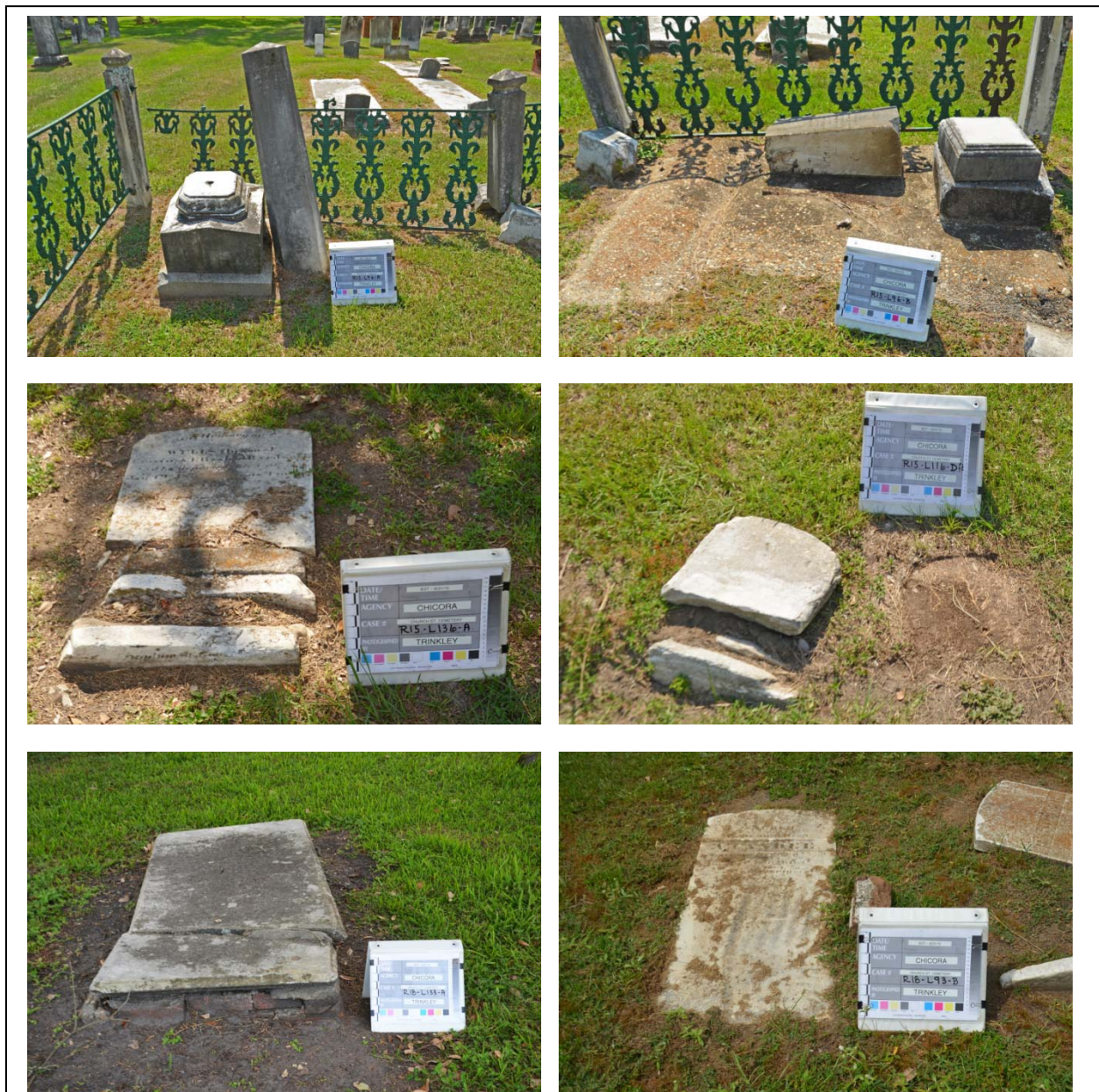
Figure 50. Types of stone damage at Church Street Graveyard. Upper left shows a fallen obelisk and tilted base that will require a tripod to reset. Upper right shows a similar obelisk that also broke when it fell and requires more extensive repairs. Middle left photo shows a tabletstone with multiple breaks. Middle right photo shows a footstone with a simple break that has been further damaged by aggressive mowing. Lower left photo shows a broken ledger that also requires repair to its brick support. Lower right photo shows a stone that may not have a base. It may be possible to provide a new slotted base for resetting the stone.
