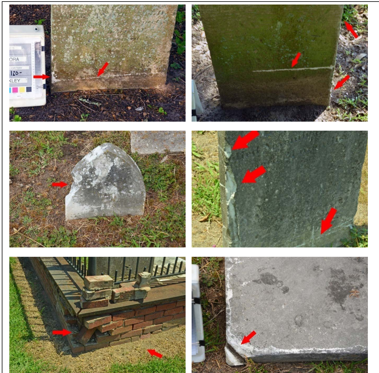
Figure 30. Mower damage at the Church Street Graveyard. Upper left photo shows a mower impact (on the left) and scrape across the reverse of a stone in R11 L120. Upper right photo shows damage to one of the stones in the Jewish section in R12, L119. In addition to the scrape, there is edge damage on the right from the upper to the lower arrow, indicating repeated strikes. Middle left photo shows a stone in R17 L84 hit so hard that a large fragment has been removed. Middle right photo shows a stone in R14 L37 with multiple impacts and multiple scrapes at the bottom. Lower left photo shows a brick wall, R4 L37, which has been so severely impacted by a mower that bricks have been not only dislodged, but also shifted to the right. Lower right photo shows a ledger in R19 L102 with the corner broken and additional mower damage along every edge.
