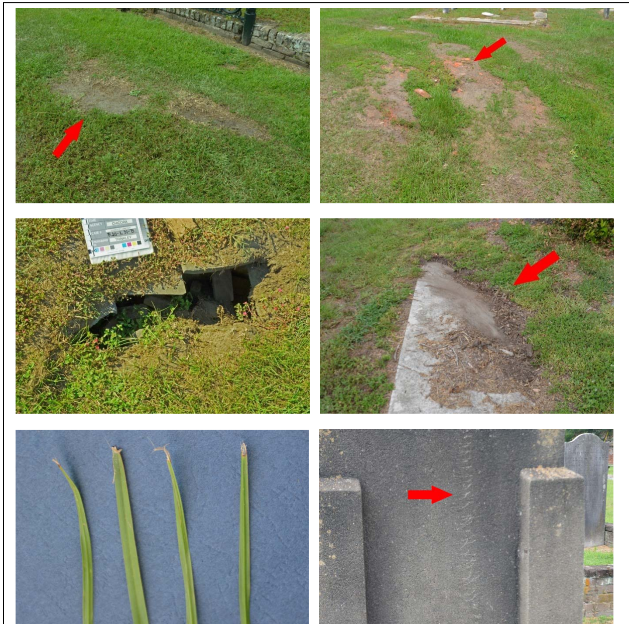
Figure 32. Other mowing problems. Upper left photo shows scalped grass in the cemetery, resulting from use of mowers that are too large. Upper right photo shows where scalping has exposed brick remains on a seemingly vacant plot. Middle left shows damage to the below ground vault resulting from a heavy mower breaking open the vault cover. Middle right shows a ledger that, while sinking, is also being covered with mowing debris never blown off. These debris are “mulching” on the marble, leading to the loss of the monument. Lower left photo shows grass tips that have been torn – not cut – by dull mowers at the Church Street Graveyard. Lower right photo shows trimmer damage up the face of a monument, probably the result of an effort to remove vines using incorrect equipment.
