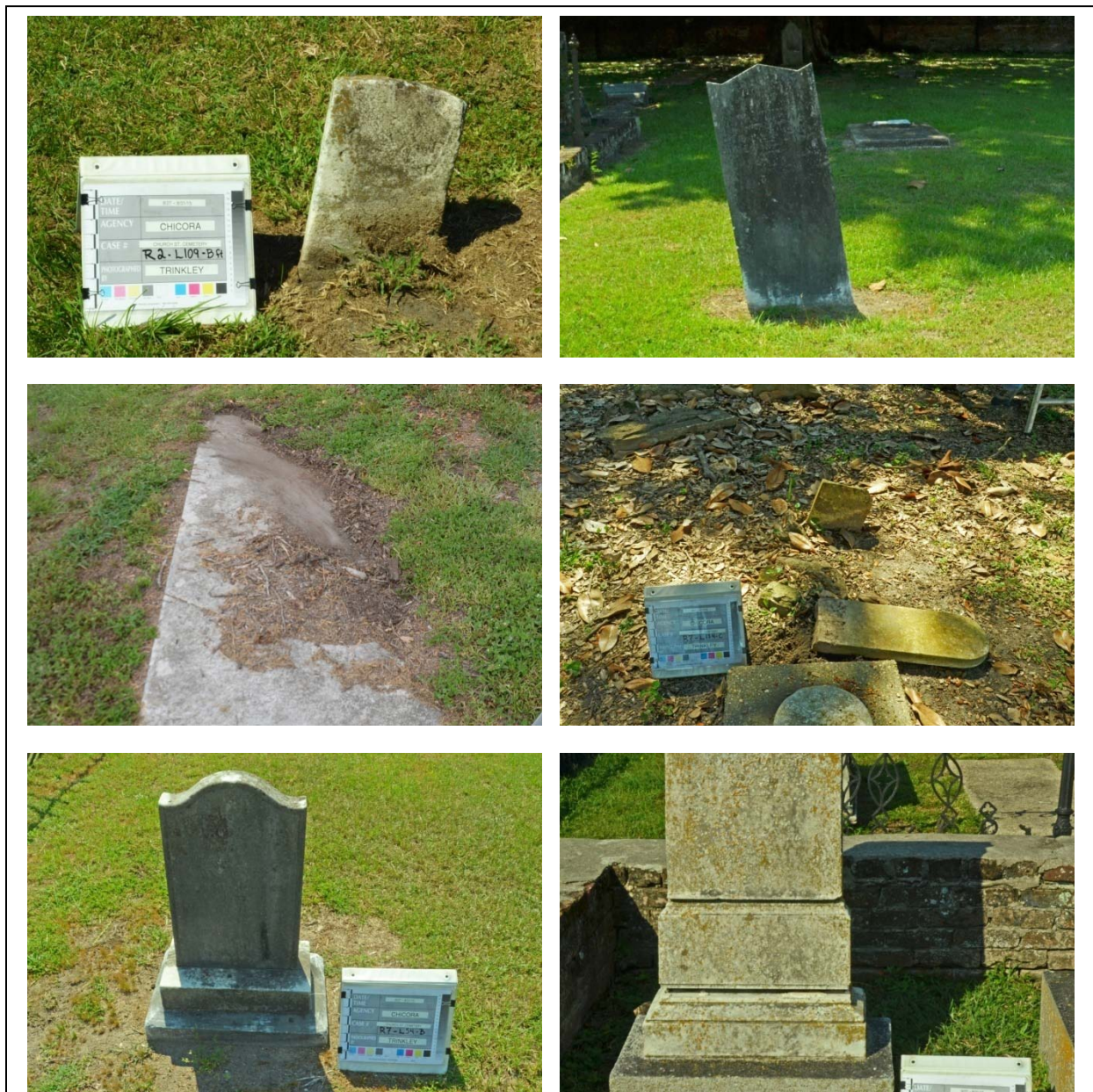
Figure 48. Types of stone damage at Church Street Graveyard. Upper left and right photos are of a footstone and tablet that require simple resetting. Middle left photo shows a ledger that requires excavation and resetting on a solid foundation. Middle right photo shows a tilted footstone in the background and, in the foreground, a footstone that is entirely out of the ground and requires resetting. Lower left photo shows a die on base monument that is both tilted and unattached, so it is unstable. Lower right photo shows a die on base monument with pins that has been shifted backward placing pressure on the pins and risking serious damage.
