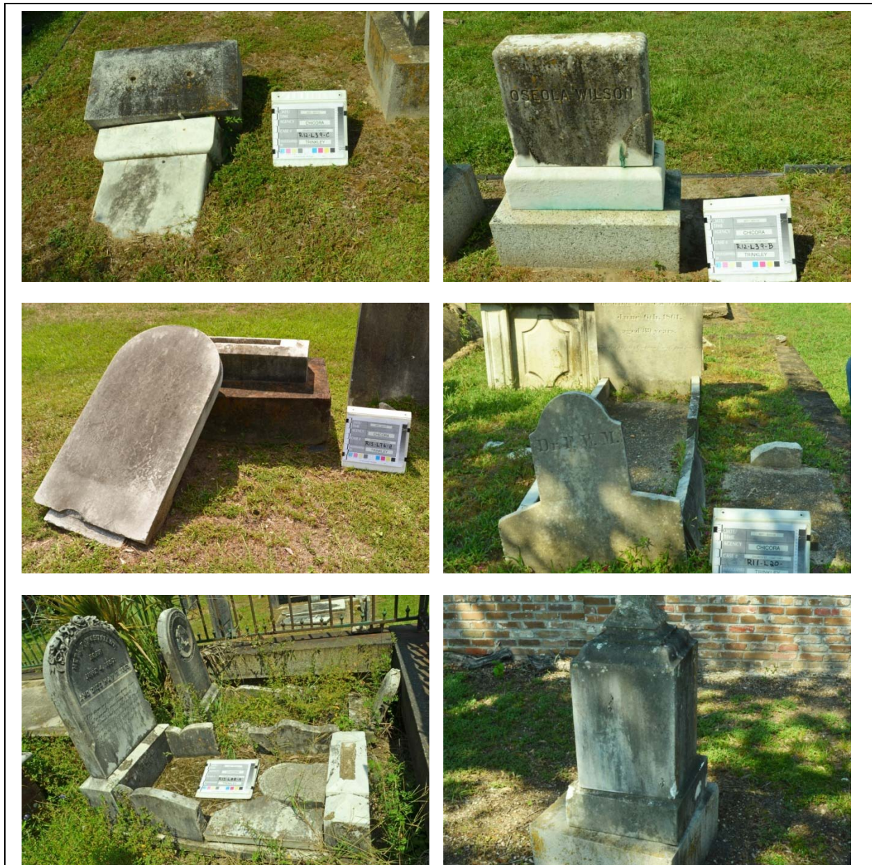
Figure 49. Types of stone damage at Church Street Graveyard. Upper left photo shows a die on base that has toppled. The original pin holes are visible in the base and one pin is shown caught between the granite sub-base and the marble base. Upper right shows a die on base that had ferrous pins. Iron jacking broke both corners. The ferrous pins were replaced by brass pins (note the staining) and OPC was used as a repair. Middle left photo shows a fallen tab in socket stone that needs only to be reset using a high lime mortar. Middle right photo shows a partially collapsed cradle grave with broken side rails. Lower left photo shows two damaged cradle graves with fallen and broken side rails and tilted or displaced dies at the head and foot. Lower right photo shows a die on base that has nearly shifted off its base because it lacks pins.
