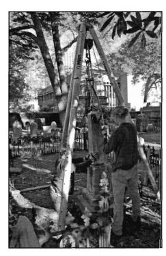
Here Chicora conservators are using a Spanco 1ton tripod to lift an obelisk into position. Instead of straps we're using a Monument Liftall, a device that can safely pick up and hold heavy stones. Note also that everyone is wearing gloves and steel-toed boots.
